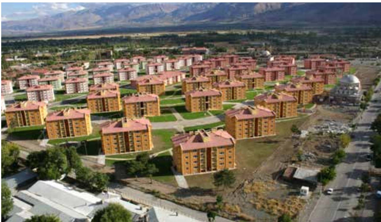
Tenure Responsive Land Use Planning is a key tool for housing and slum upgrading projects. Urban renewal project in Turkey. © UN-Habitat
