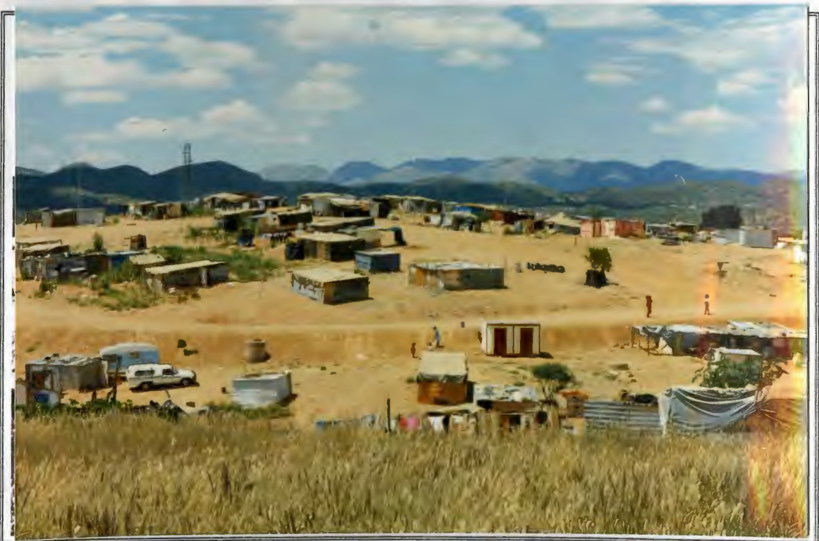
Completed infrastructure works is also seen from the Onghuuo ye Pongo Oshatotwa Community Centre, looking at the Onyeka community. Graveled community streets and a sewage pipe access manhole are seen in the centre (along with the communal water tap and toilets)
