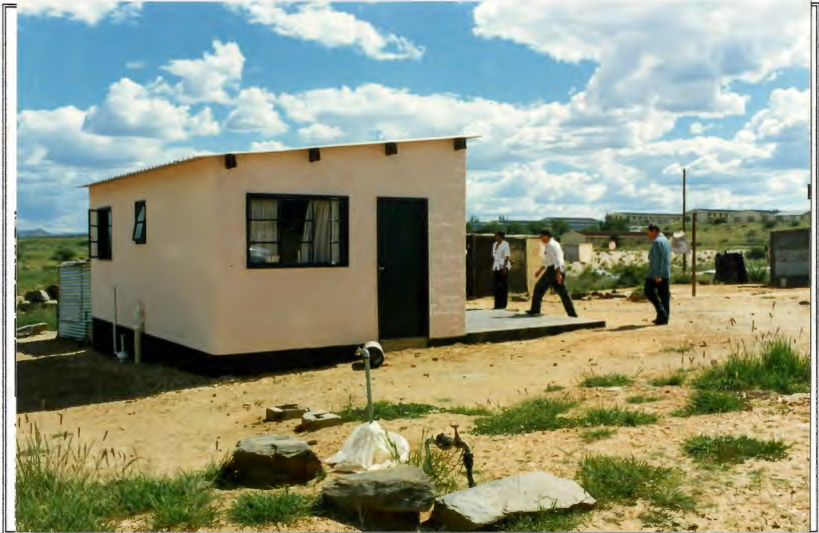
The first house completed as a starter solution within the Upgrading Project is this two-room unit belonging to Mr. Reinhold Amushelenga, of Freedomland. CDC Ms. P. Taaru, Oshatotwa Chief Technical Advisor, Mr. J. A. Crispo, and Mr. Kenneweg from the German Embassy are shown visiting the house in February.
