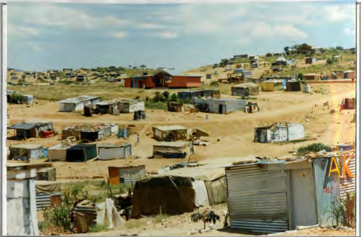
Infrastructure work has been completed in the eastern areas of the Upgrading Project. Here the Onghuuo ye Pongo Oshatotwa Community Centre is shown with a completed street below it. Note the municipal equipment, just to the right of the Centre, preparing the main street for tarring
