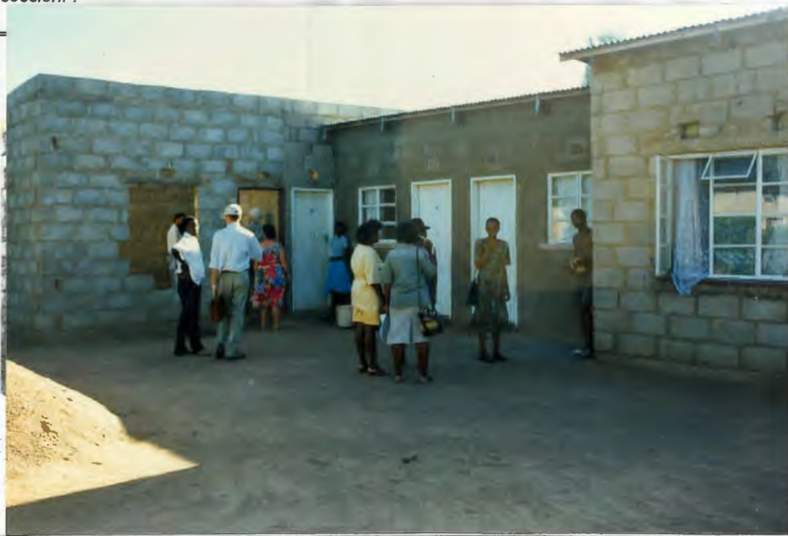
Ten members of the Oshatotwa team took a Study Trip to Botswana in early March, visiting low-income housing projects in Gaborone and Kanye. Here members of the team and hosts from the Botswana Christian Council inspect one SHHA compound where incremental building is evident. The first unit was the two-door central building, built with a loan from BCC. The additional wings were built - and expansion continues - with the owner's personal investment
