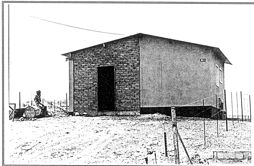
The new owners at Otjomuise have already begun improvements most of their houses. Here at erf 44 the owner has nearly completed the addition of two new rooms at his own expense.
