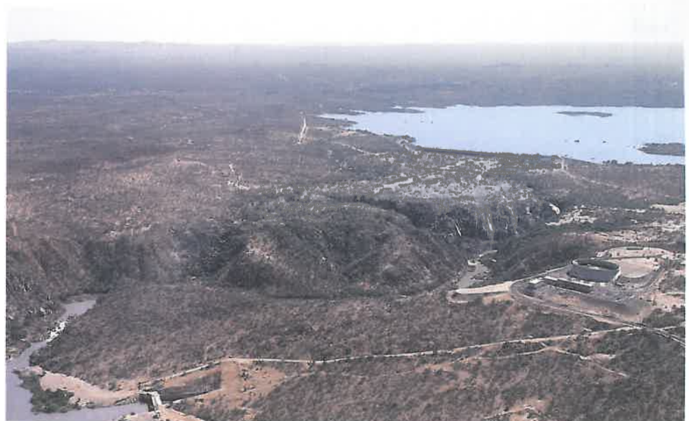
Calueque Dam was built in the early 1970s on the Kunene River just north of the Angola–Namibia border to regulate the flow of water to the hydroelectric scheme at Ruacana Falls, and to store water to be fed into the canal and pipeline system serving north-central Namibia
