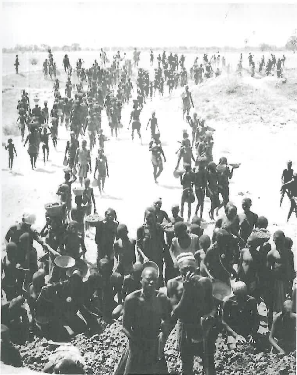
The labour of thousands of people was engaged to excavate dams during the 'Famine of the Dams' between 1929 and 1931
