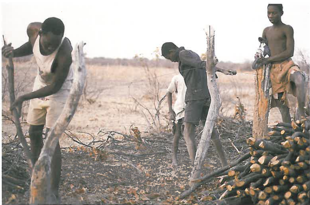
Freshly cut poles being added to a new fence
