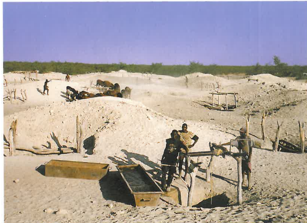
Each well in this group of hand-dug wells (oondungu) is owned by a different family. Buckets are lowered on long ropes to draw water lying 20–30 metres below the surface.
