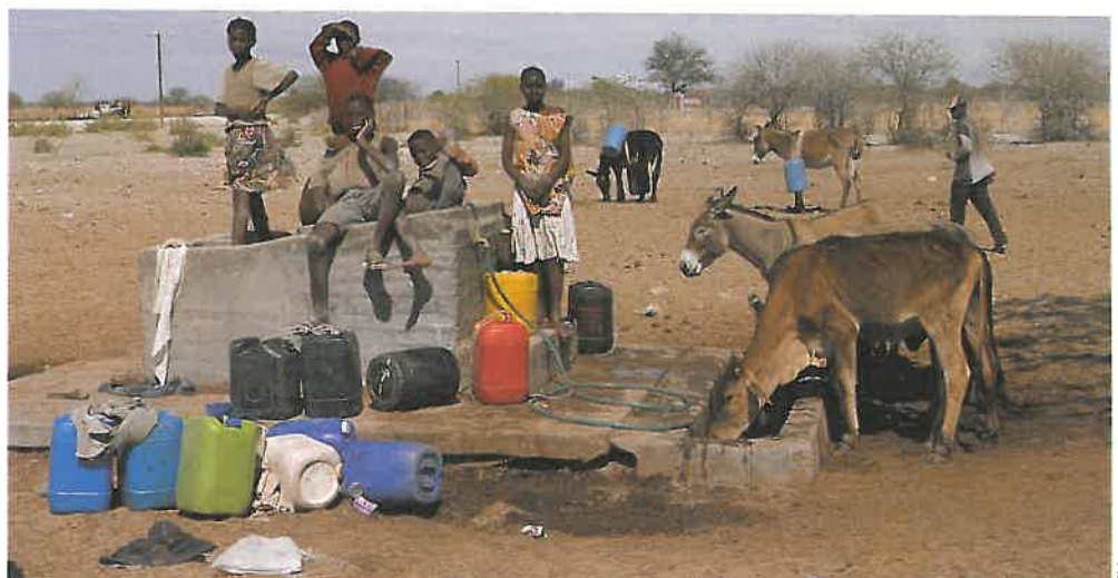
One of thousands of water points along the network of pipelines
