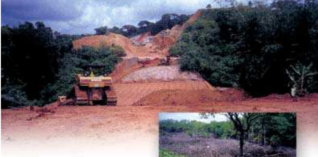
A section of the Compact Road under construction in Babeldaob, Palau, 2002.
