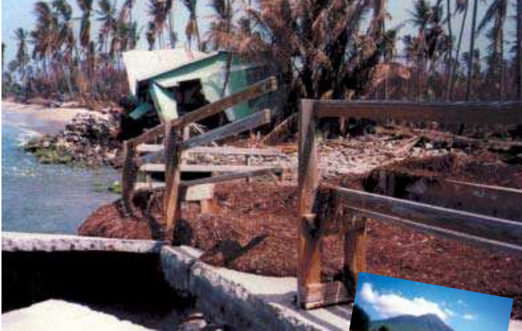
Damage at Pinney's Beach, Nevis, after Hurricane Luis in 1995.
