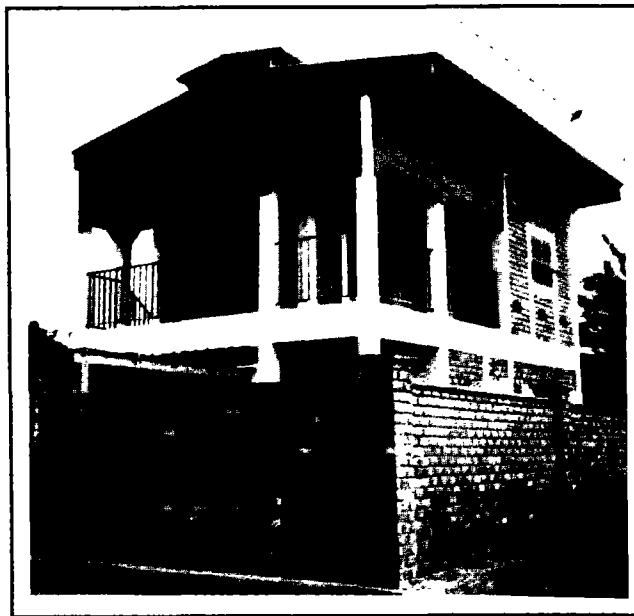
A key part of VITA's Djibouti energy strategy is the promotion of energy-conserving alternatives in private, government, and industrial buildings. The project has assisted construction of several energy-efficient 'bioclimatic' building designs. These include dispensaries and low-cost housing units built from cheap, locally-available materials. Pictured above is the 'Chef de Quartier' home, which, built from Djibouti-made fired bricks, does not require air conditioning to remain cool in the searing heat common to Djibouti.
