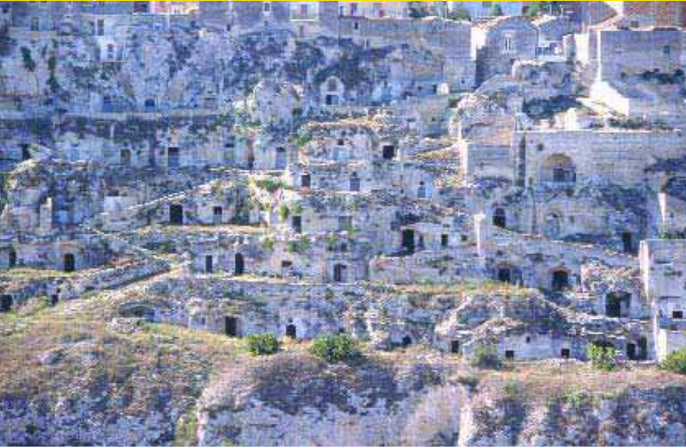
Photo 3. The roofs are part of the stone work; not a single drop of rain is lost. © Pietro Laureano
