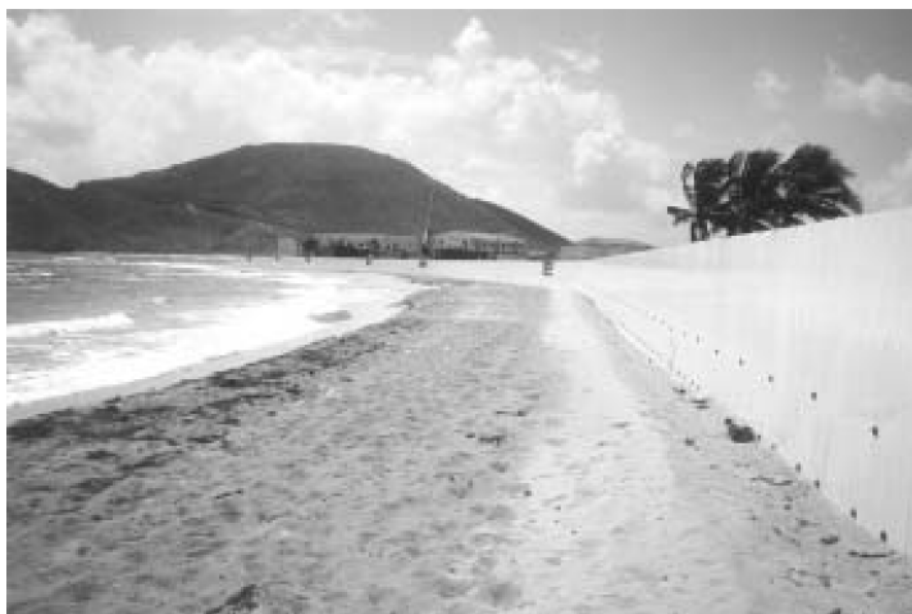
Photo 9. Seawall at North Frigate Bay, St Kitts. February 2000.
