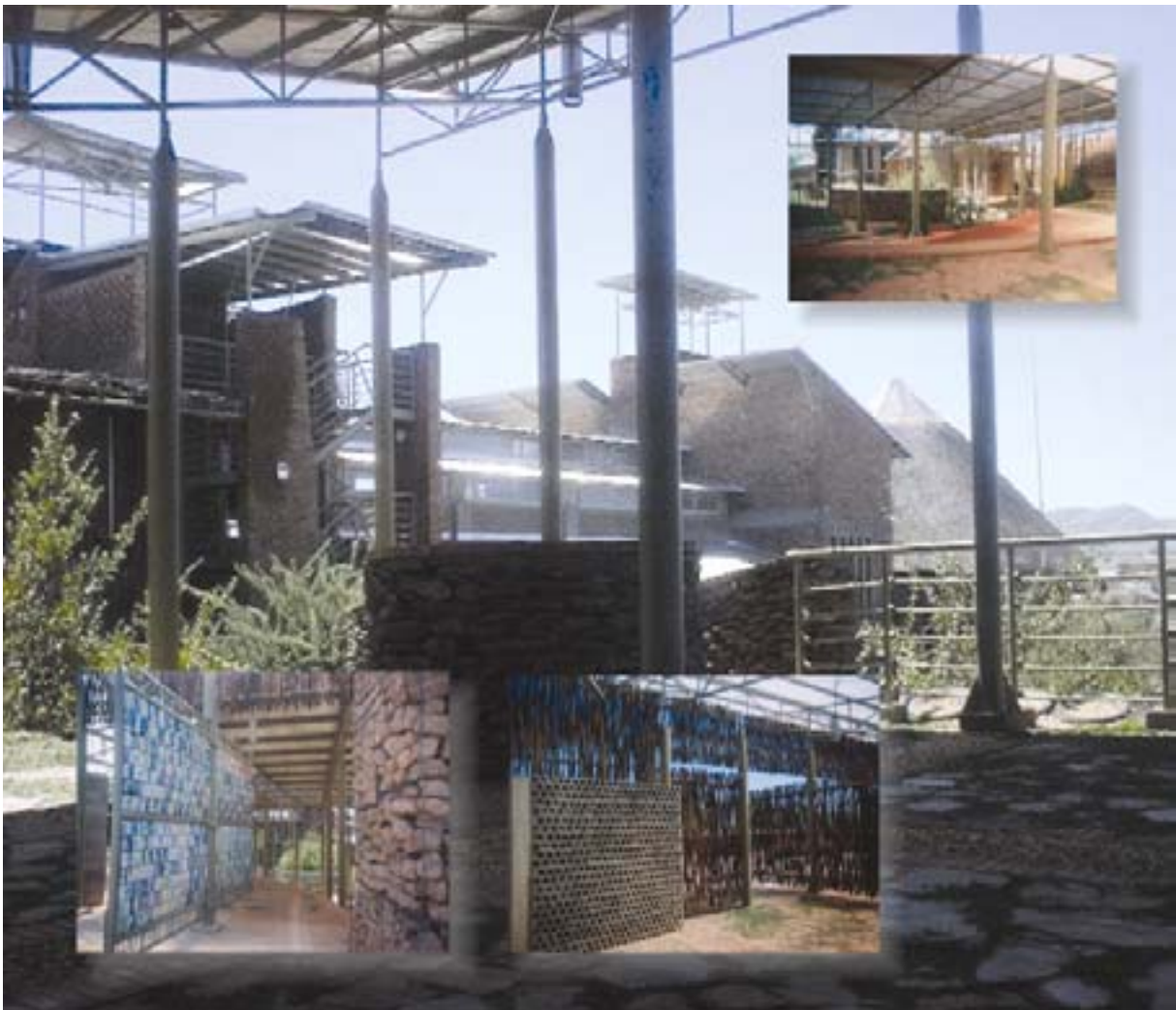
The UN Habitat Research and Development Centre in Katutura is built almost entirely from alternative low-cost materials such as clay and car tyres, and serves as an excellent example of what can be achieved with such materials.
