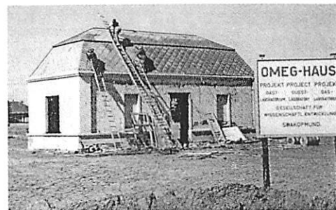
Omeg House during restoration.
