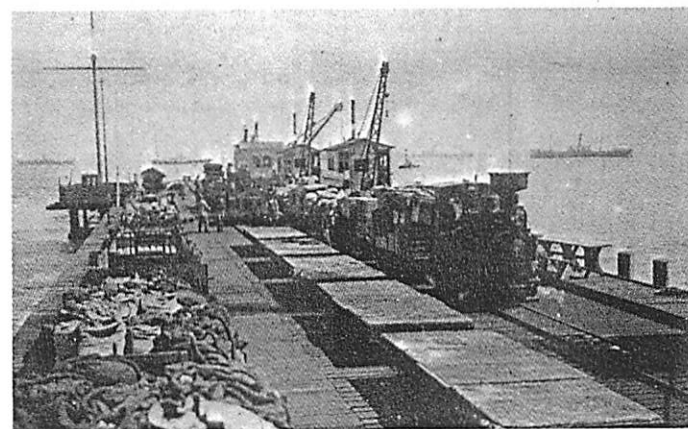
Removal of offloaded goods from the wooden jetty.
