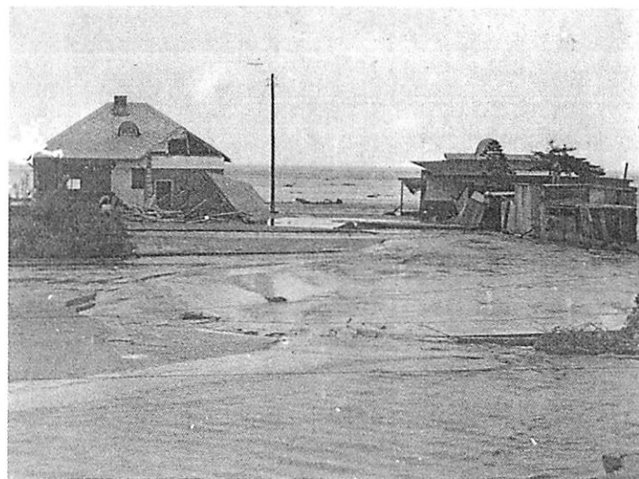
Devastation caused by floodwaters of the Swakop river, 1934.
