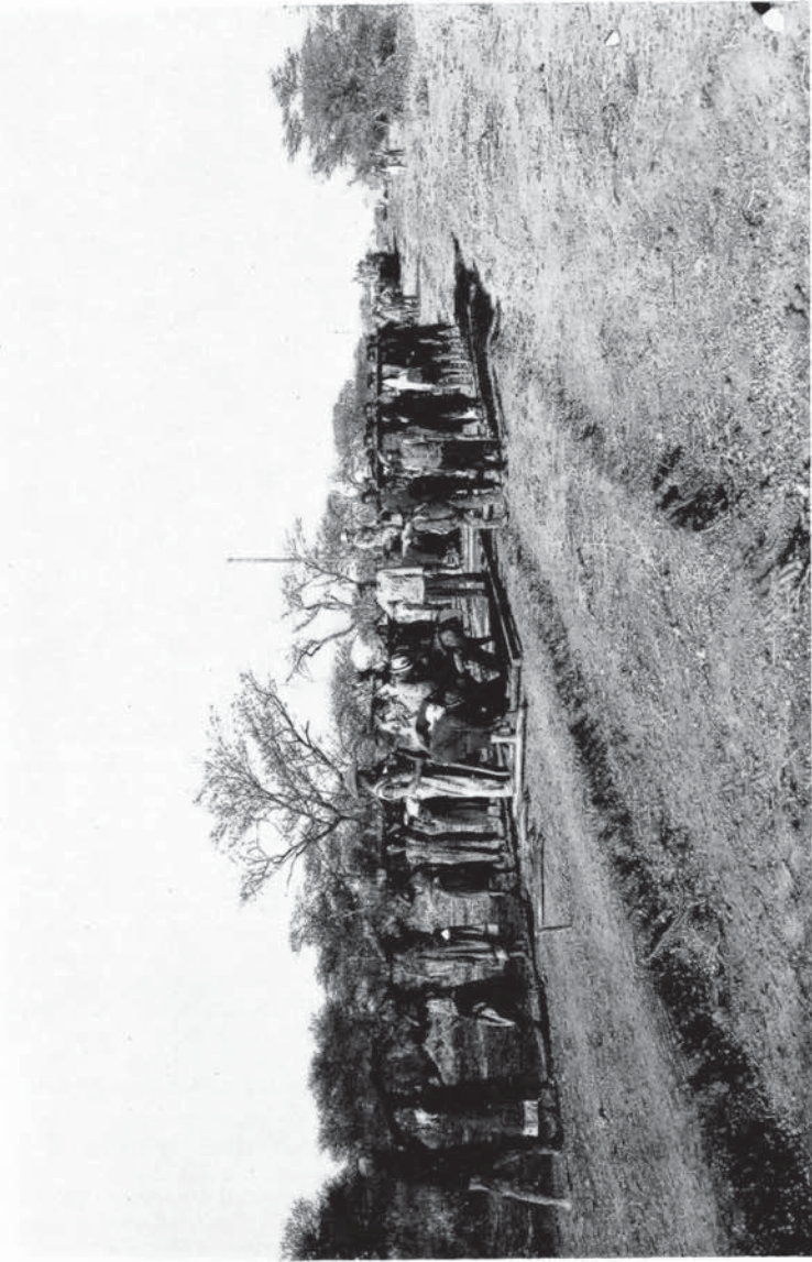
PHOTO 3: Labour gang on railroad construction between Otjiwarongo and Tsumeb, 1905. Note native women carrying steel sleepers on their heads. (Collection: W. Schatz)
