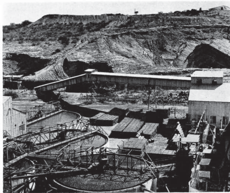
PHOTO 23: View across part of concentrator showing thickener tanks, stockpiles of flotation reagents and abandoned fillwaste cuts on Huetttenberg. (Alice Mertens, 1961)
