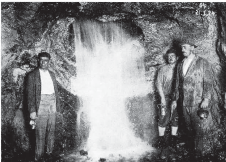
PHOTO 11: Water gushing from cavity in Tsumeb mine, January, 1924. Director F. W. Kegel (left) and Mine Foreman W. Klein (right). (O.M.E.G. collection of photographs)
