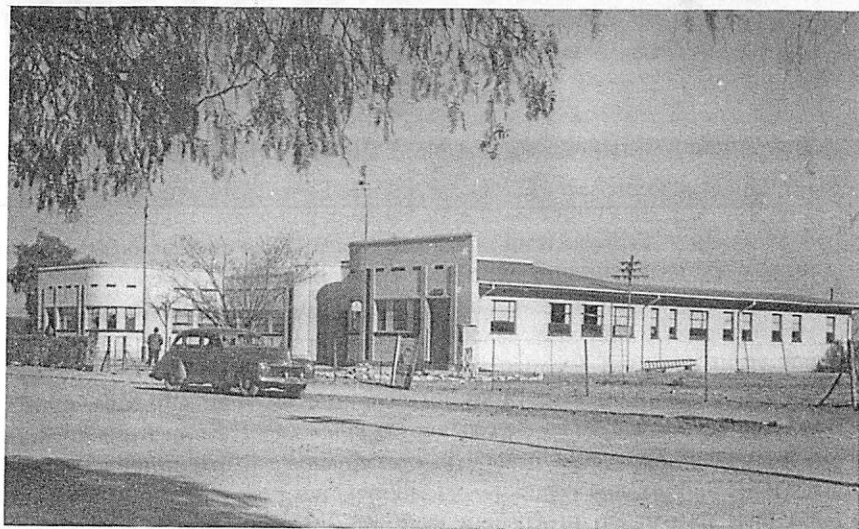
Complex housing the post office, police station and magistrate
